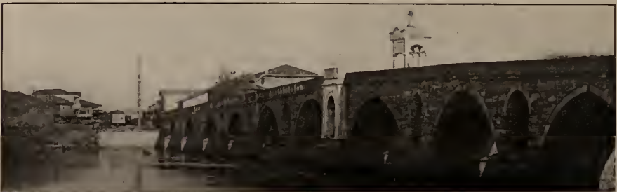
THE BRIDGE OVER THE MARITZA RIVER, NEAR ADRIANOPLE
